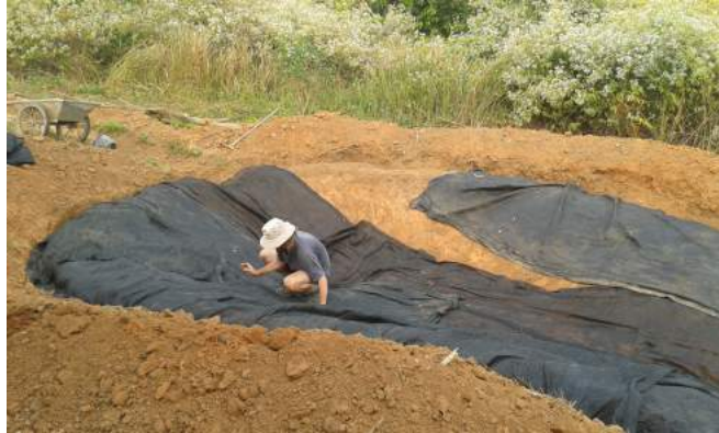
Lining a pond with plastic liner and shade cloth in Kailash Akhara, Thailand
