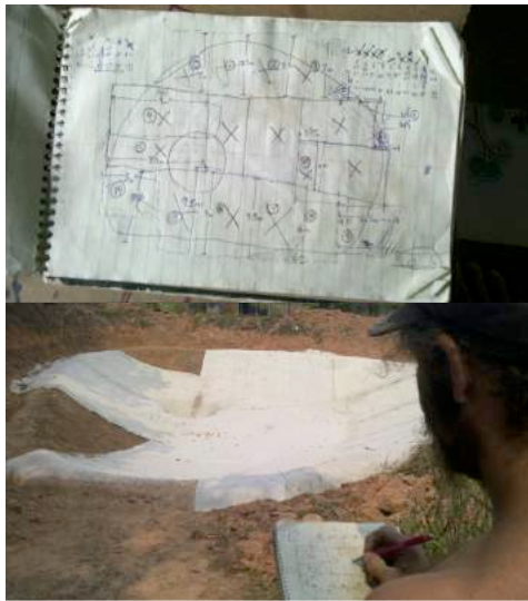
Pond liner installation, Panya Project, Chiang Mai, Thailand. This sketch (left) indicates where different lengths of bentonite liner need to be cut and set in place (picture on right has about half of the strips set in place)
