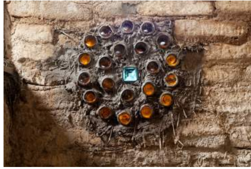
Glass bottle wall, set in cob, in-between adobe earth bricks Panya Project, Thailand
