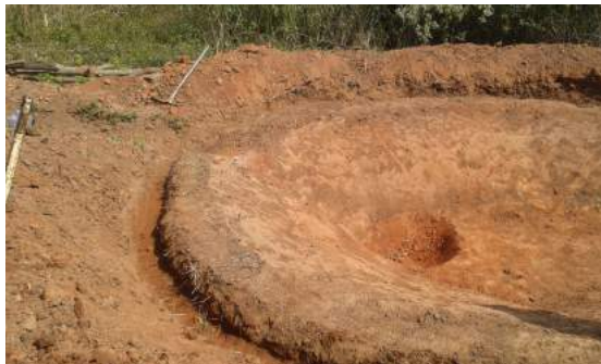
Digging a "shelf" at the top of the pond provides a space to tuck the plastic liner.
