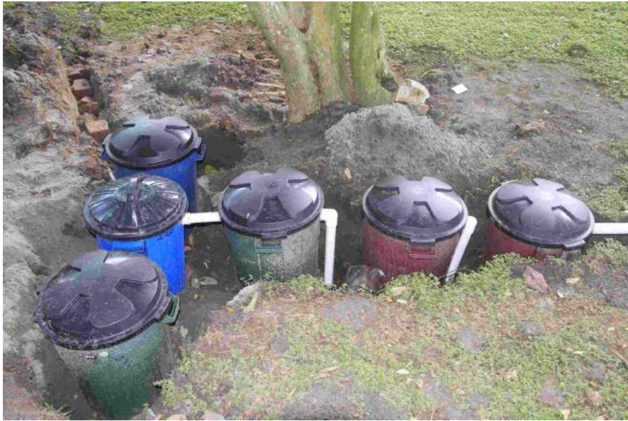
Bucket grease trap (source online)
